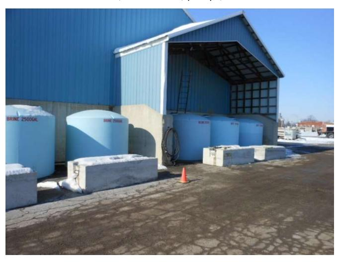
Electric 1 ½" 2HP Pump to Blend Tanks with Beet Juice and Salt Brine Fill Trucks
