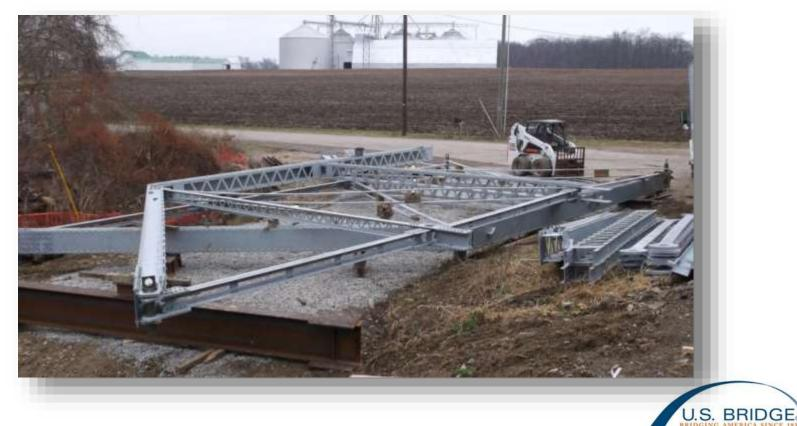
Reinstallation began with carefully placing and anchoring the support frames on the Liberty.
