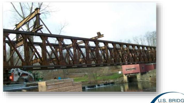
The pre-assembled end sections were placed on the support frames.
