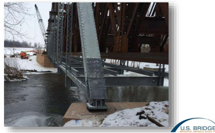
Another flood caused zero interruption. The new stringers and wood floor was installed with the Liberty still in place.
