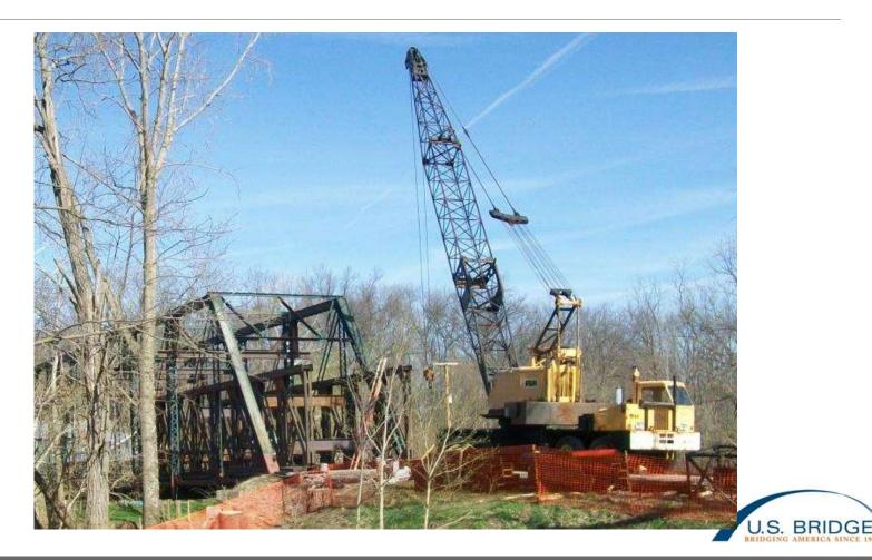
The Hillman rollers were placed under the Liberty bridge on a steel channel so it could be rolled across the existing deck.
