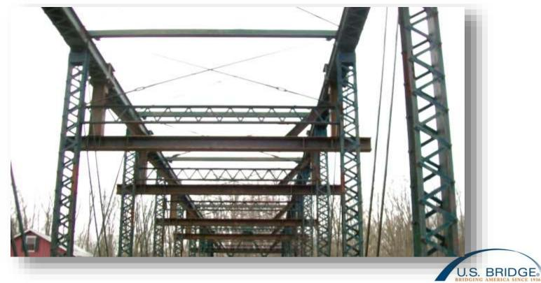
Frames were bolted to top chord so that lift points would release dead load stresses in the bottom chord and tension diagonals.
