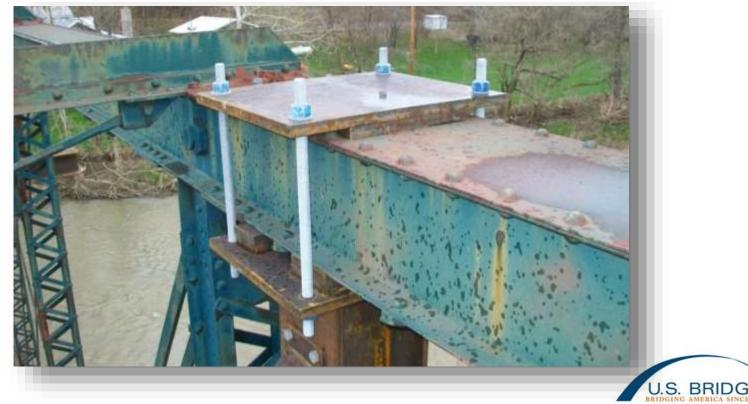
Framework was constructed to establish pick points below the existing Portal Bracing.
