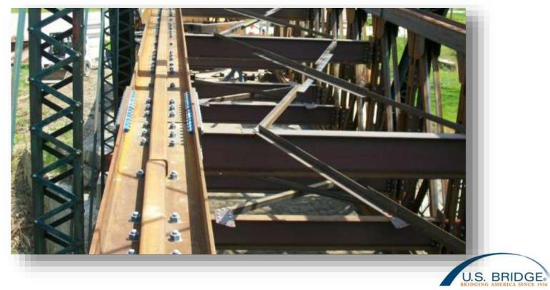
A tubular rail was used to space the rollers away from the bolted connections of the Liberty.
