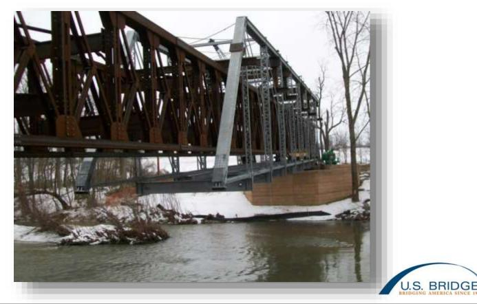
Unequal sag of the Liberty and uniform camber of the Indian Mill truss was accommodated with shims between the rollers and the support frames
