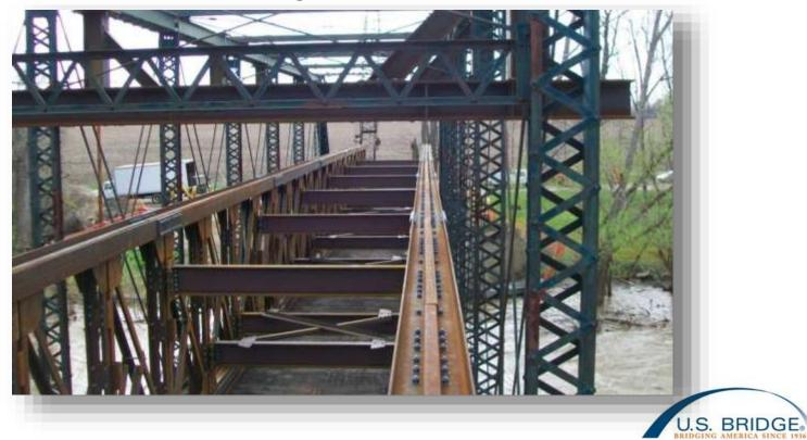
The Liberty floorbeams were staggered at top and bottom connection points to create additional top chord bracing.
