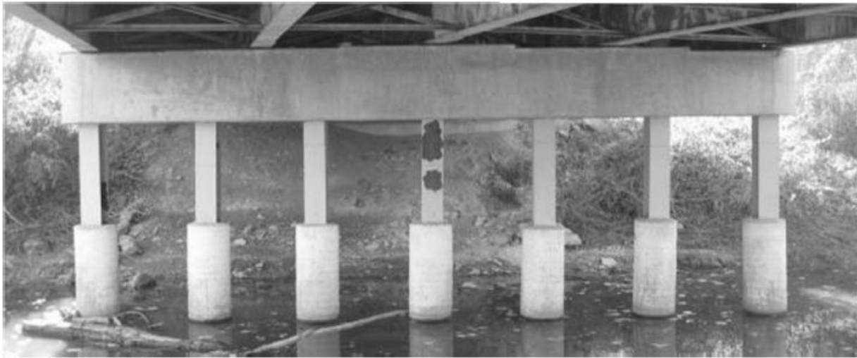
Figure 93 - Capped Bile Bent
