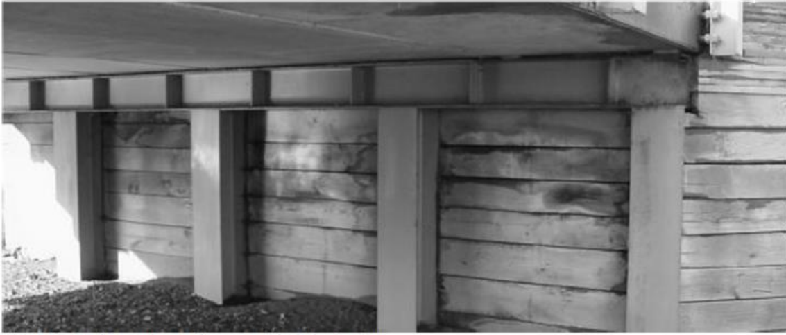
Figure 91 - Steel Capped Bent Abutment with Timber Lagging
