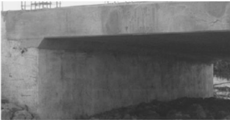
Figure 87 - Stub Abutment
