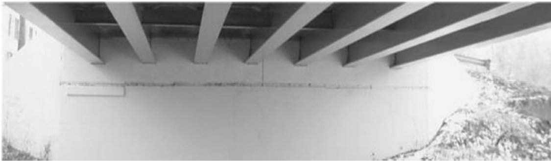
Figure 88 - Semi-Integral Abutment
