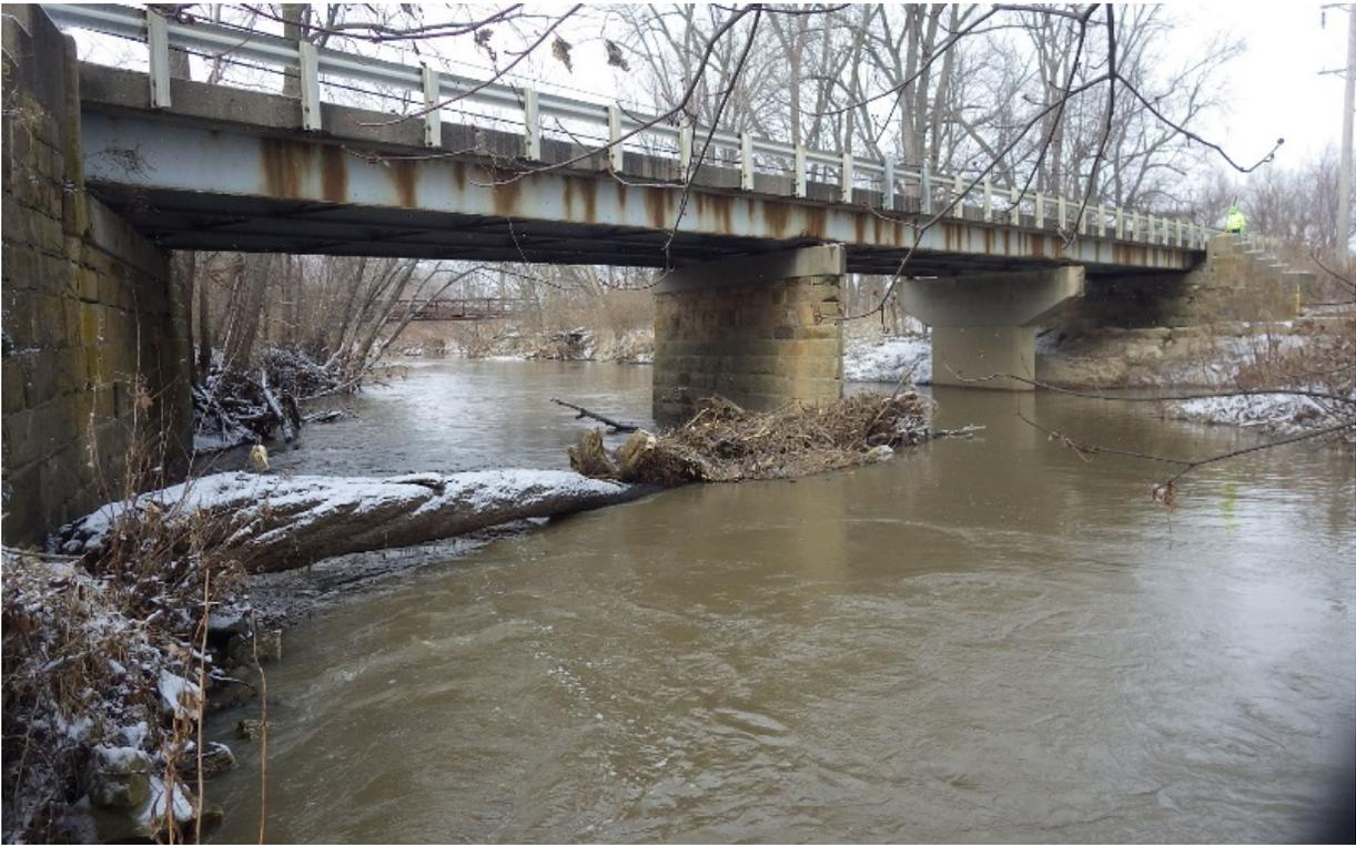
*Figure 8- Good Example of Baseline Photo Looking Downstream from SE Corner (Best Downstream Option)*
