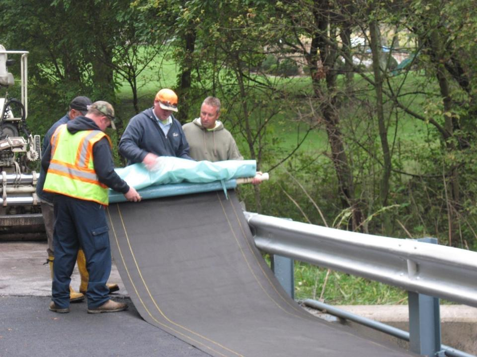
Waterproofing membrane (geo-tac) is "sandwiched" between two layers of asphalt concrete. (2" thick at edge and 5" thick at center) The material cost is about 70 cents per square foot.
