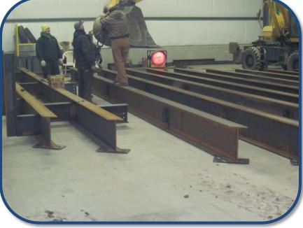
EACH BRIDGE IS COMPLETELY ASSEMBLED THEN DIS-ASSEMBLED BEFORE BEING GALVANIZED. THIS BRIDGE HAS 11 W18X55 BEAMS AT 2.6 FT. SPACING AND WILL BE COVERED WITH A TIMBER STRIP DECK WITH WATERPROOFING AND A VARYING ASPHALT THICKNESS FROM 2"-5".
