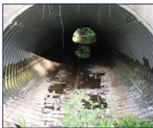
Corrugated Metal pipe prior to repair
