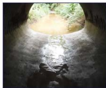
Pipe after gunite rehabilitation
