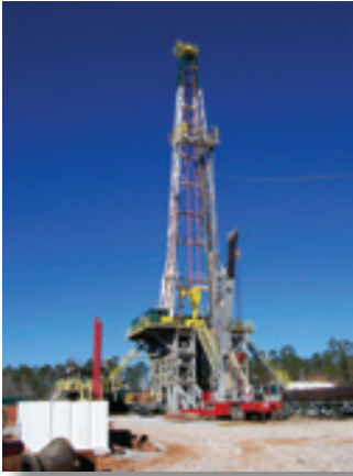
Well drilling rig
