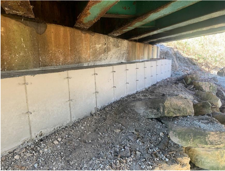
Scour has been encapsulated and remediated
