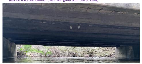
Item 60 Substructure.......8 Agreed Again, without having to access the abutments physically, I could not sound the abutment faces. There is a fair amount of staining and water leakage, but no spalling. Given the age a visual appearance, age and efflorescence where the curb line falls, I would rate this abutment a 7.
