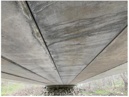
The beams have unusual horizontal shear cracking that appears to have initiated during, or shortly after construction. It appears to be stable and not a structural issue, having been there for the best part of 20 years. It is unknown if the interior beams have this condition. The manual does not address this type of cracking. I could go with a 6 or 7 on the superstructure. I lean toward a 7 due to the condition of the beam bottoms, including the fascia beams.
