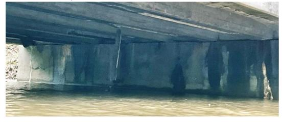
Item 61 Channel......8 Agreed While the channel looks to have a good alignment, a tree has recently fallen across the channel upstream of the bridge and has the potential to cause scour to develop.
