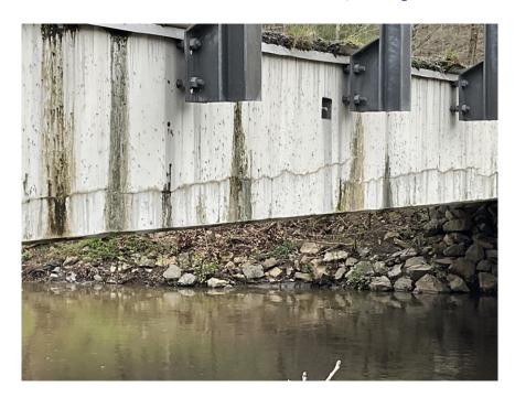
Item 60 Substructure....... 8 There is some cracking along the top of the abutment along the beam seats about 4 inches down. I would rate this a 7 for that reason.
