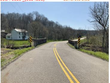
This is coded as a Slab bridge, but it a through girder bridge, as the main reinforcing steel runs laterally from girder to girder and not along the centerline. Hopefully the load rating is based on what is in the girders as well as the slab.
