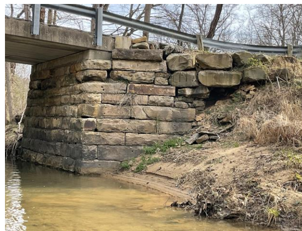
Item 61.01 Scour..6 Agreed Flow line up against abutment, but no apparent exposure or undermining detected.
