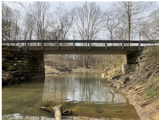
Item 61.01 Scour..6 Agreed Flow line up against abutment, but no apparent exposure or undermining detected.
