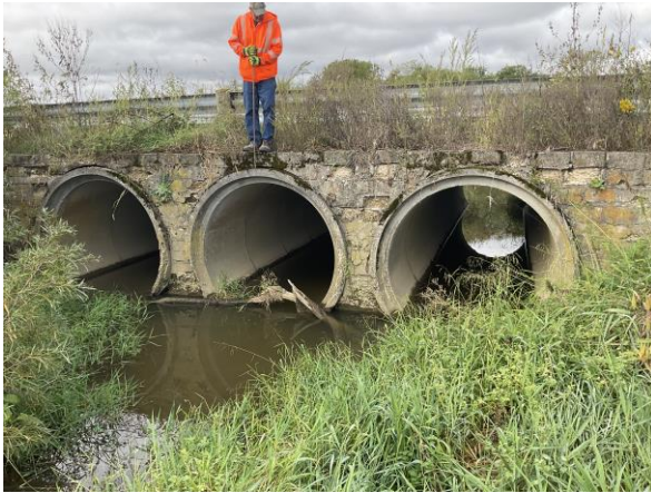
Defect Photos: None Channel Photos: Good Channel Photos
