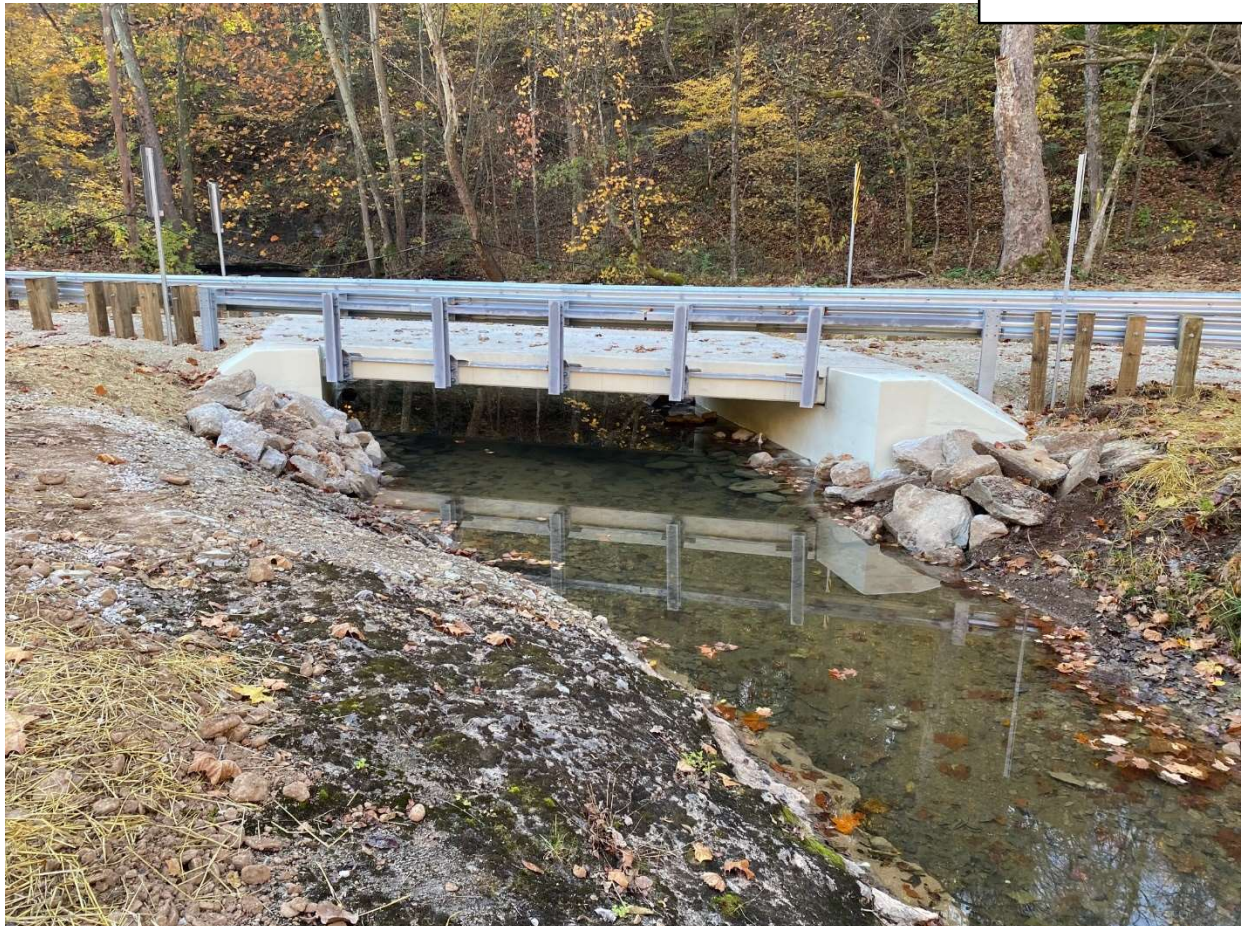
TR1206-0.01 Bridge replaced in 2024
