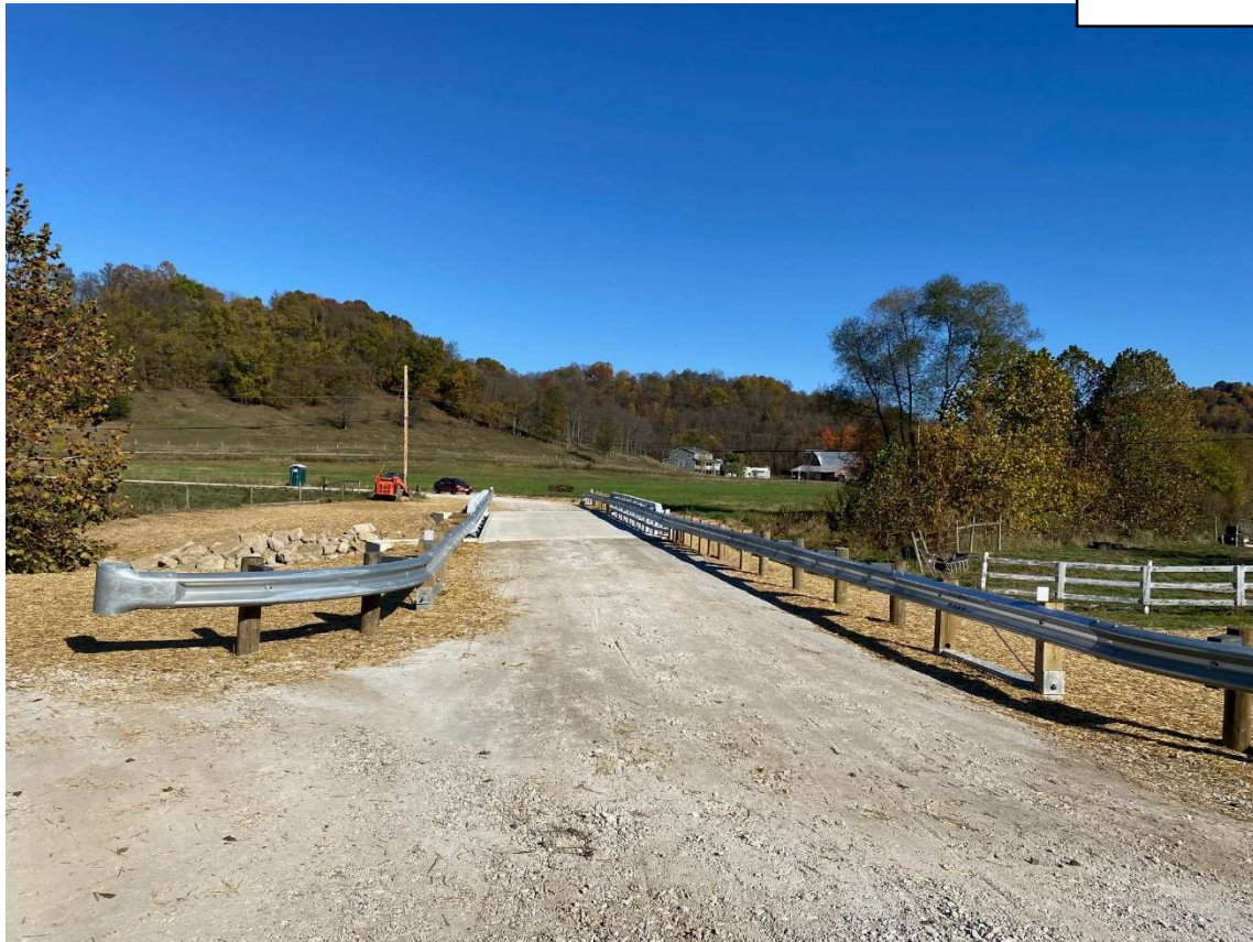
TR2001-0.13 Bridge replaced in 2024
