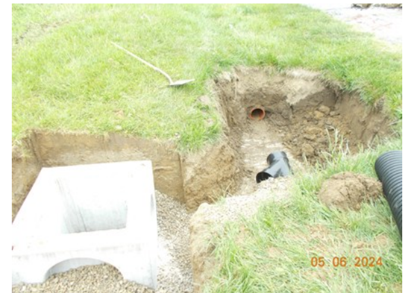
To the left is an example of a drainage tile main replacement. To the right is a catch basin relocation/replacement. Both projects were completed in 2024.
