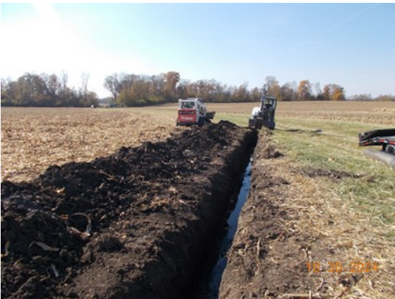
To the left is an example of a drainage tile main replacement. To the right is a catch basin relocation/replacement. Both projects were completed in 2024.
