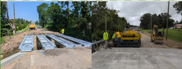
CLI-CR15-5.78 Gurneyville Rd Bridge
